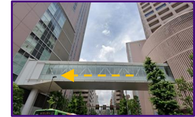
Skywalk Bridge (Walking from Bldg. No.1, 2 nd Floor)
